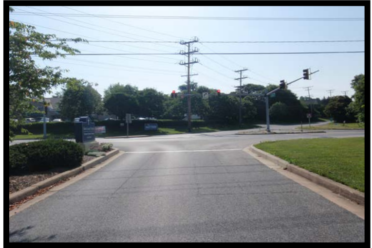
SB Entrance to Church at MD 108
