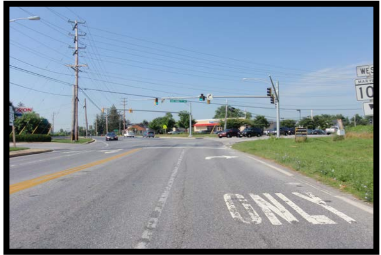
WB MD 108 at Ten Oaks Road / Gas Station Entrance
