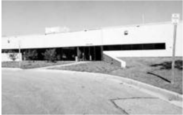
Howard County Detention Center
