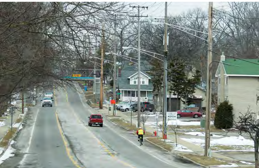
Figure 7. Addition of a Bike Lane Creates a Buffer between Pedestrians and Moving Vehicles Photo Credit: Jennifer Atkinson
