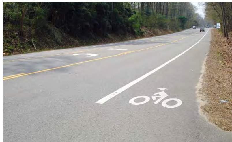
Figure 19. Bicycle Lane on Rural 3-Lane Section, Lawyers Road, Reston, VA Photo Credit: Virginia DOT
