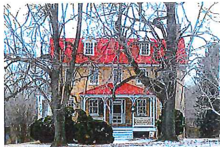
MONTROSE, CLARKSVILLE – stone masonry, red metal roof, roof dormers, hipped roof porch
