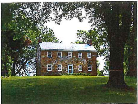
IVY HILL, MARRIOTTVILLE – masonry, gable roof, divided-lite windows
