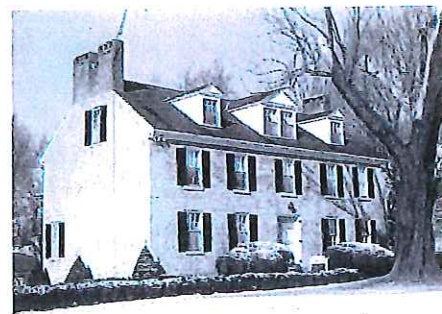
WALNUT GROVE, CLARKSVILLE – stone masonry, gable roof, roof dormers
