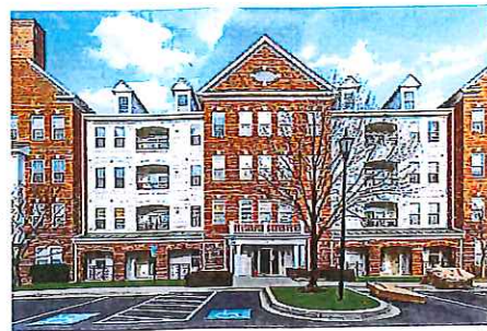
THE VILLAS OF RIVER HILL, CLARKSVILLE – brick masonry and siding composition, roof dormers, metal roofs
