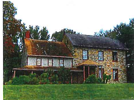
CARROLL COUNTY HOUSE – masonry and siding, window surrounds, gable roof
