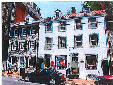
ELLCOTT CITY – masonry and siding, window surrounds, metal roof, roof dormers
