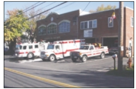
Figure 1-7, Elkridge Fire Station
