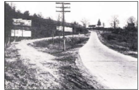
Figure 4-8, Dead man's curve, realignment in the 1930s, when Route 1 was among the most dangerous roads in the US.
