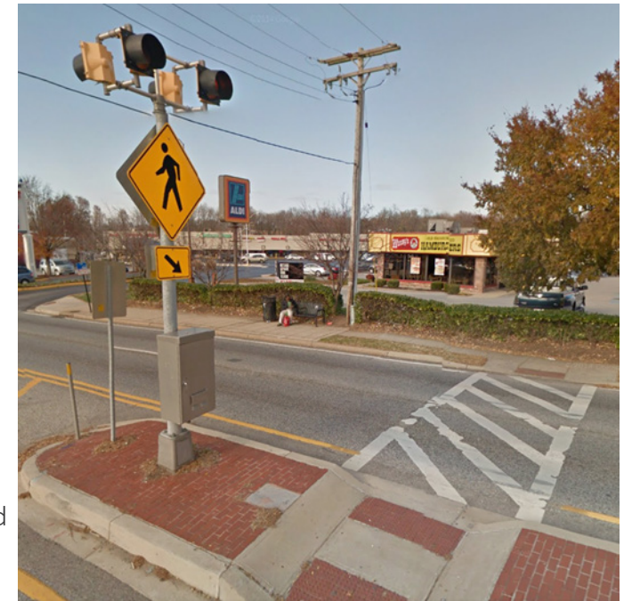
Median Pedestrian Refuge Implemented on MD 26
