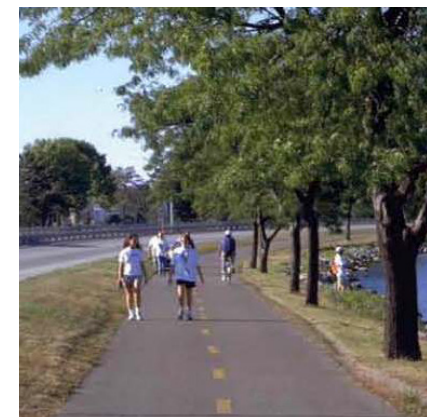
Example of a Shared Use Path from Bike Howard- Bicycle Facilities Visual Glossary page 35
