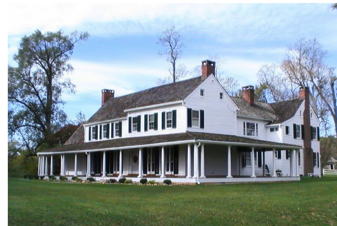
RICHLAND, CLARKSVILLE – white lap siding, gable roofs, divided-lite windows
