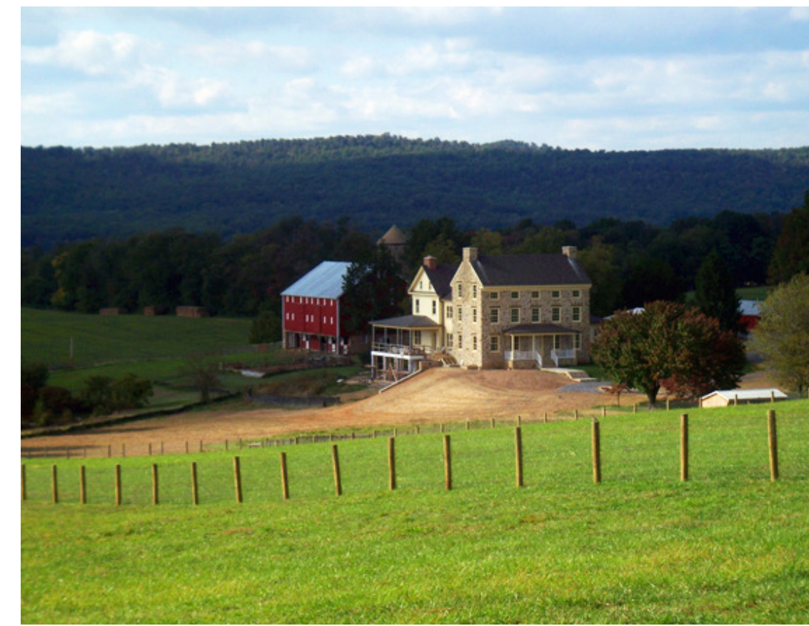
hipped roof porches, masonry and siding
