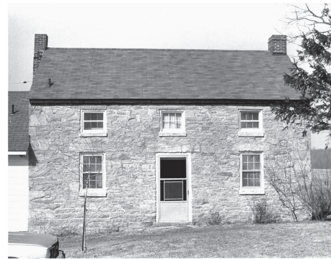
LIMESTONE VALLEY FARM STONE TENANT HOUSE, CLARKSVILLE – stone masonry, gable roof, divided-lite windows
