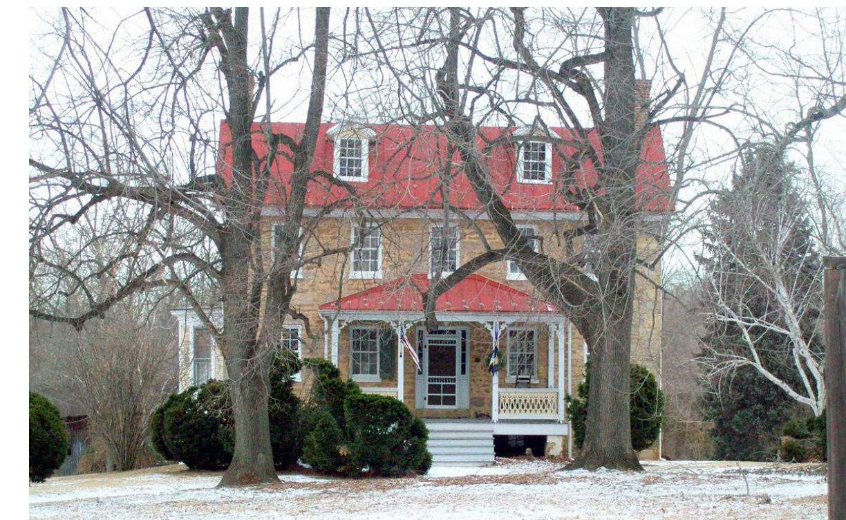
MONTROSE, CLARKSVILLE – stone masonry, red metal roof, roof dormers, hipped roof porch
