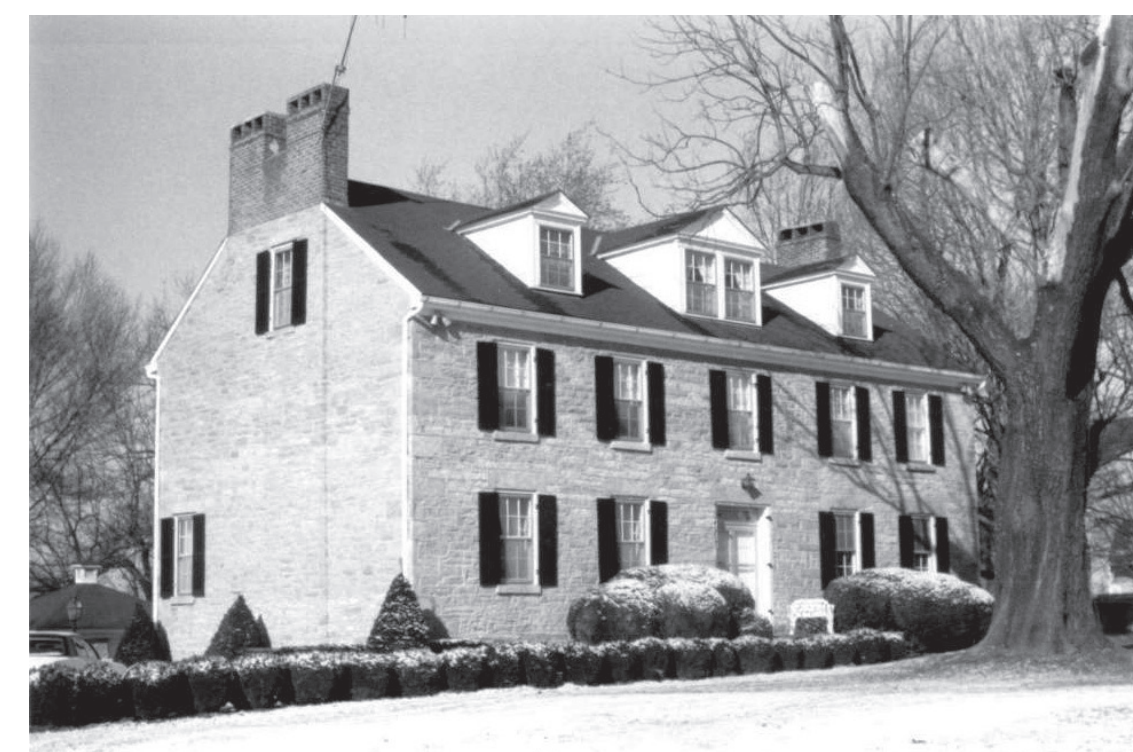
WALNUT GROVE, CLARKSVILLE – stone masonry, gable roof, roof dormers
