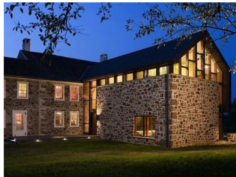
stone masonry, clerestory windows
