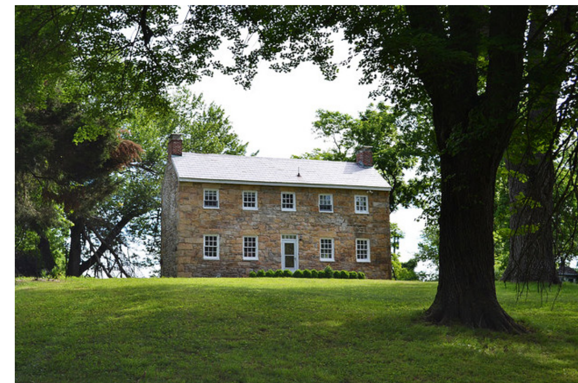
IVY HILL, MARRIOTTSVILLE – masonry, gable roof, divided-lite windows
