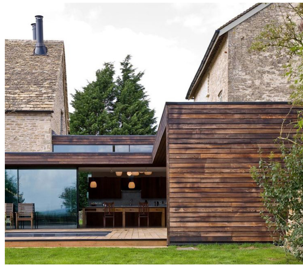
stone masonry, modern wood addition to historic stone buildings
