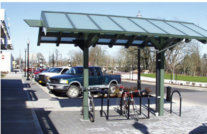
Covered Shelter Bicycle Parking
