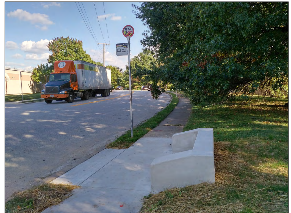
This landing pad and knee wall at an RTA bus stop on Ridge Road in Ellicott City provide an ADA-compliant place for transit users to wait for the bus.
