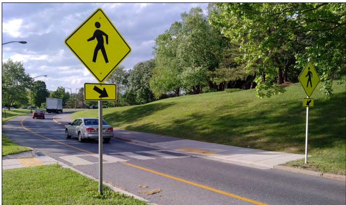
This pedestrian crossing at Broken Land Parkway and Snowden River Parkway has ADA-compliant perpendicular curb ramps.
