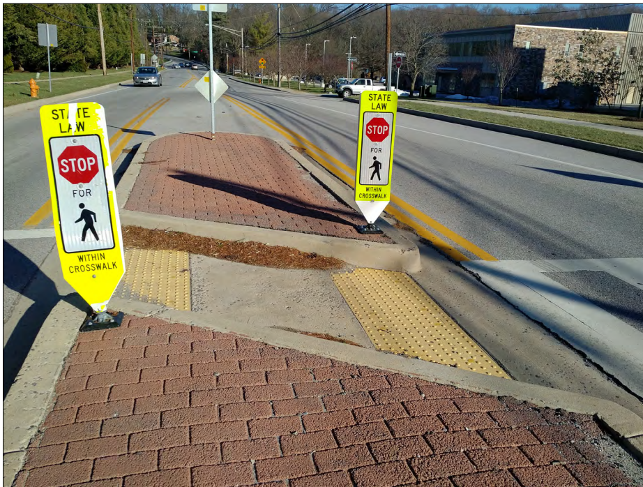
This pedestrian refuge island allows pedestrians to more safely cross Frederick Road to access the Miller Branch Library in Ellicott City
