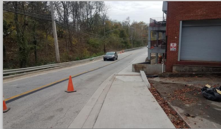
Foundry Street Pathway
