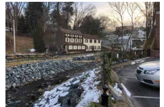
Figure 48: Daylighted Section of the Hudson Branch in Lot F
