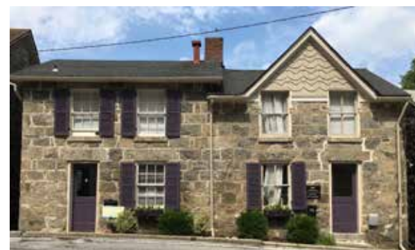
Figure 27: Rehabilitated Tonge Row Facades as part of Howard County Facade Improvement Program
