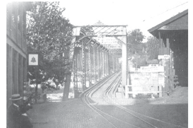
Figure 119: Historic Photo of Trolley #9 Bridge, Credit: Baltimore County Public Library/MD Covered Bridges
