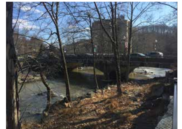
Figure 120: View to River and Main Street Bridge from Lot B
