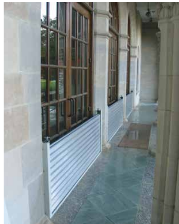
Figure 42: Non-structural Floodproofing Can Mitigate Flood Impacts, Credit: PS Flood Barriers
