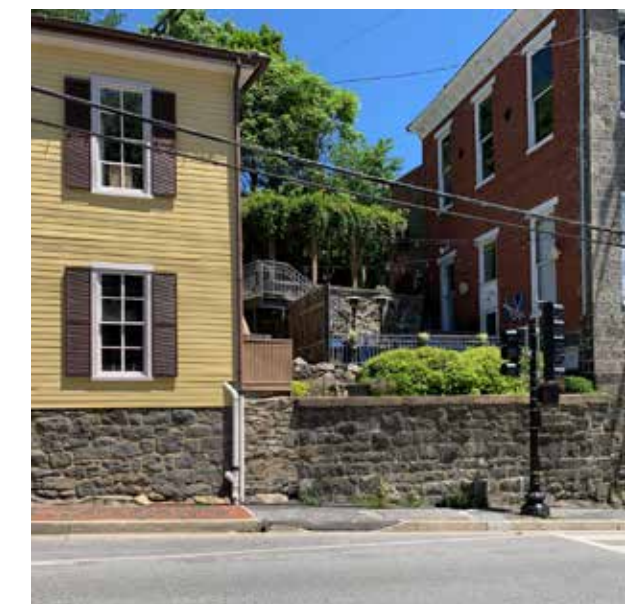
Figure 20: Typical Materials of Mid-19th Century Buildings in Ellicott City Include Stone, Brick and Wood Frame
