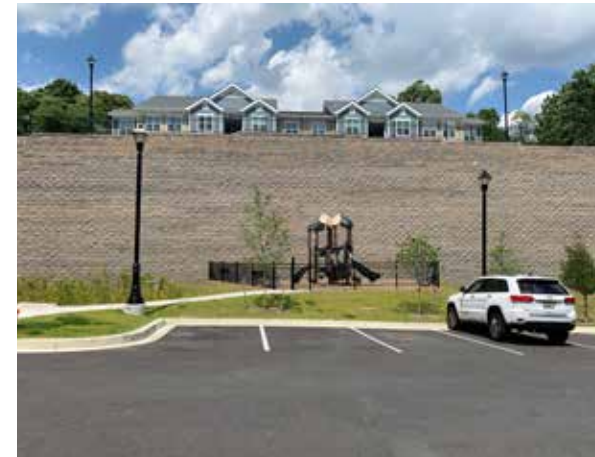
Figure 24: Architecture Not Responding to Overall Site
