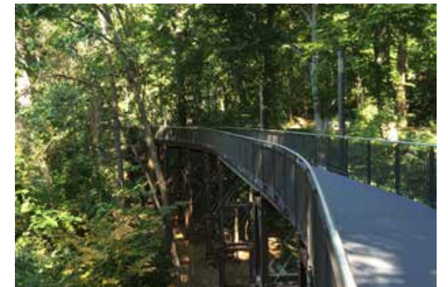
Figure 80: Pedestrian Bridge through Trees, Johns Hopkins, Baltimore, MD
