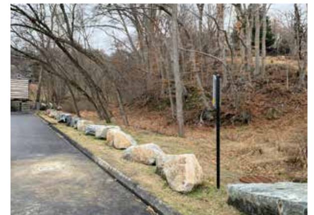
Figure 181: Existing Constrained Tributary East of Lot F
