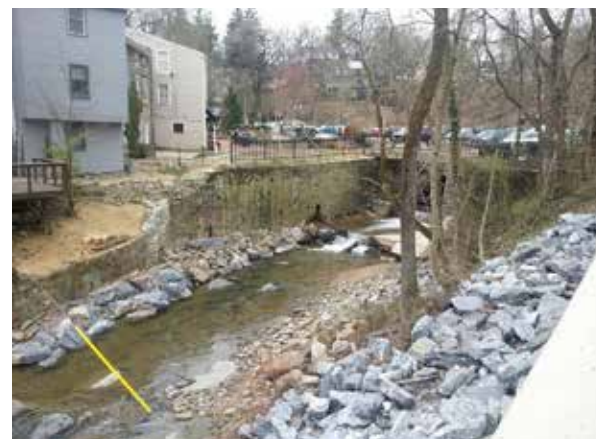
Figure 155: Hudson Branch along Tonge Row and Hamilton Street
