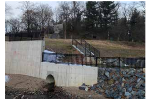
Figure 47: Existing Culverted Stream Outfall in Lot F
