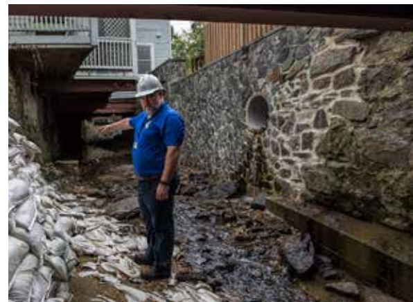
Figure 144: Character of Existing Stone Channel Walls
