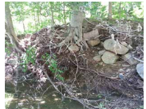
Figure 38: Vulnerable Tree Cover Along Stream Edges Creates the Potential for Debris Mobilization and Damage Downstream
