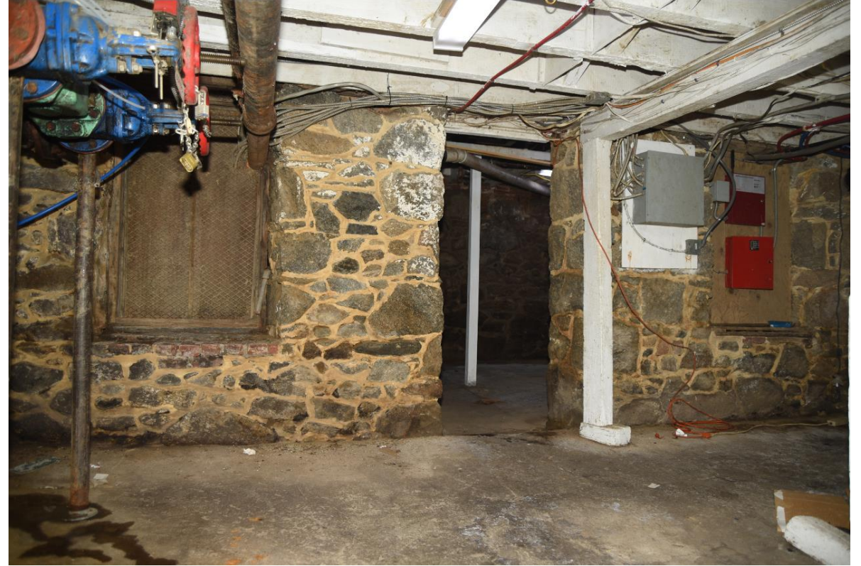
South wall of basement, on interior.
