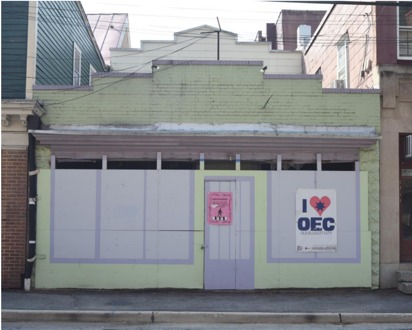
8055 Main Street front facade Commonly known as Discoveries Photo date 8.25.2020
