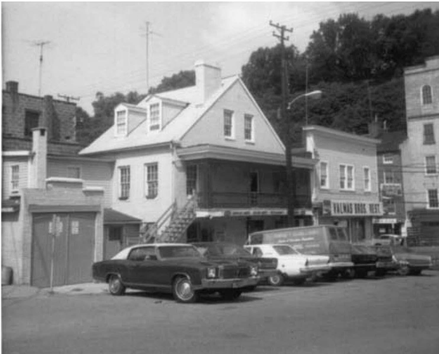
8049 Main Street - Rear and east side of building along Tiber Alley and Maryland Avenue
