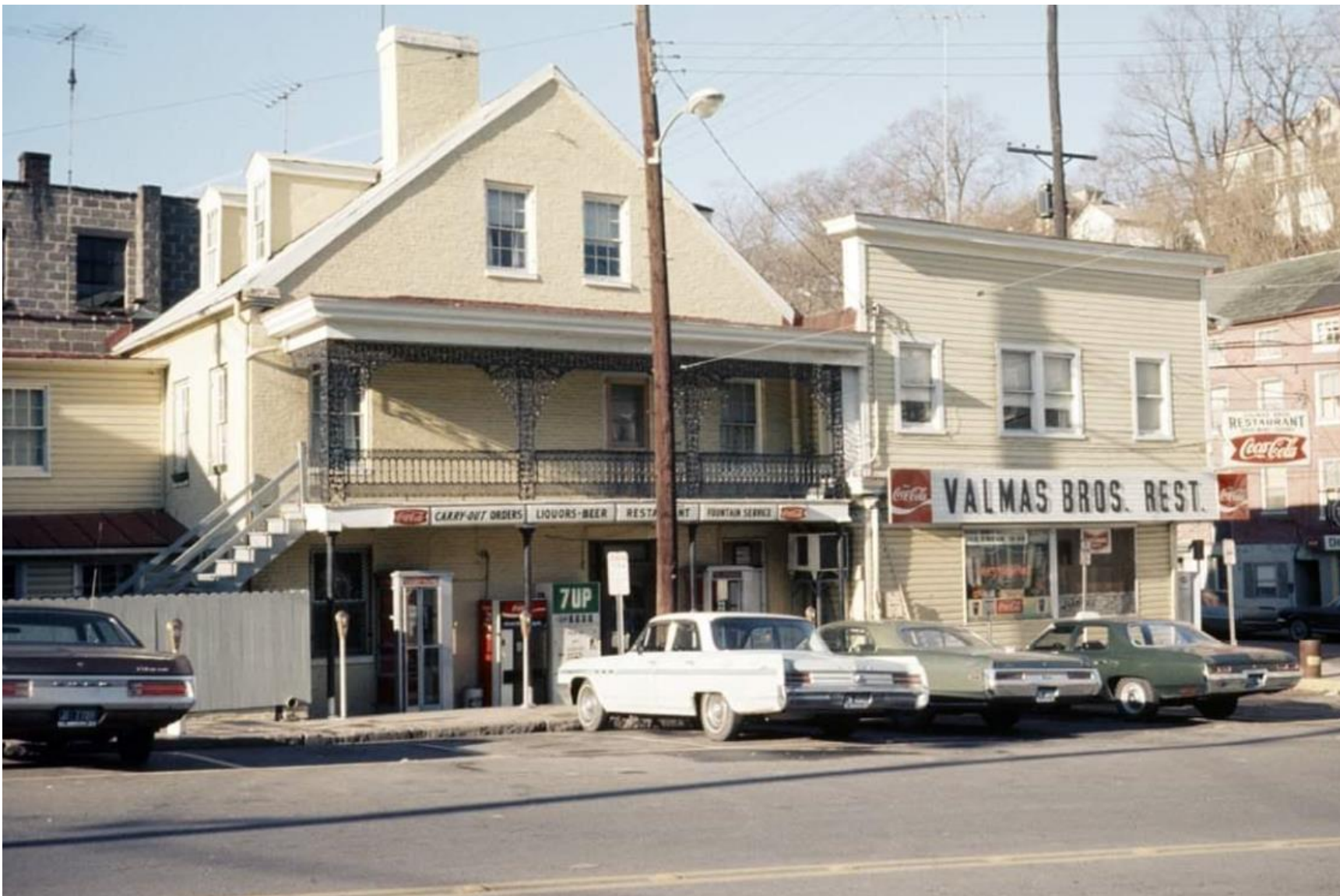
8049 Main Street - East side of building along Maryland Avenue
