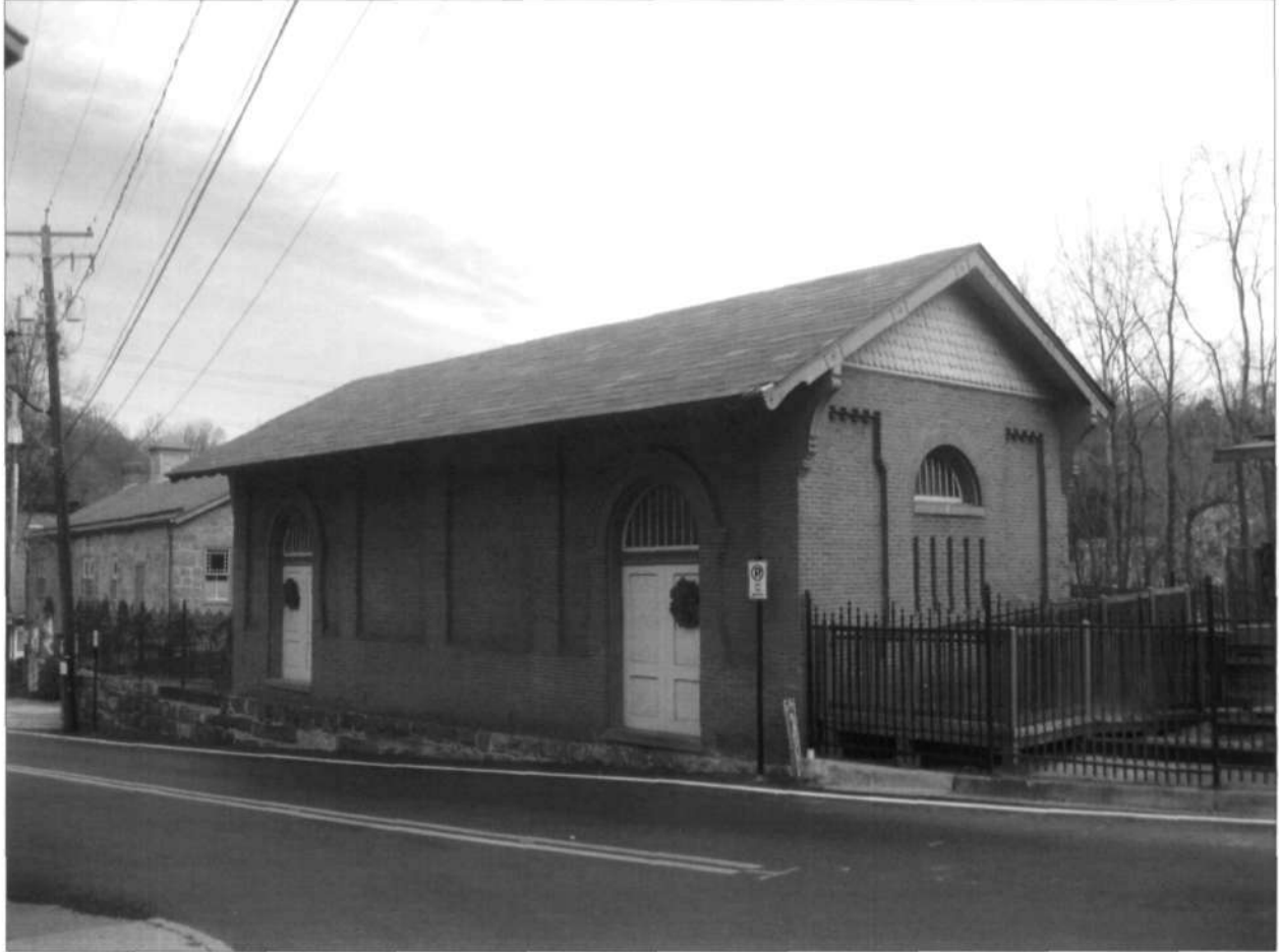
HO-71 Ellicott City B&O Railroad Station, Freight Building, and Turntable 2711 Maryland Avenue, Ellicott City Photos by Jennifer K. Cosham, 12/5/2012 Freight building, southwest elevation
