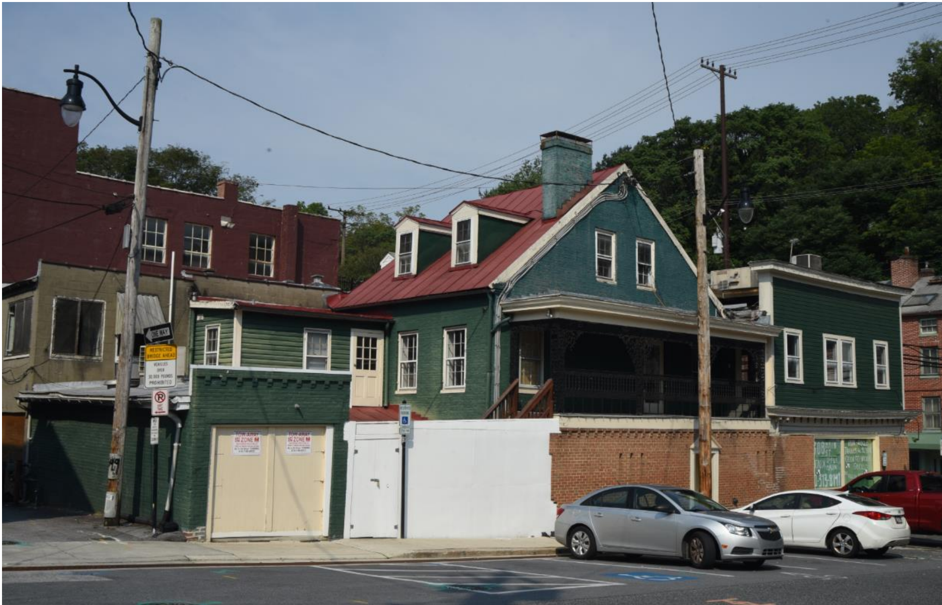
8049 Main Street - Rear and east side of building along Tiber Alley and Maryland Avenue
