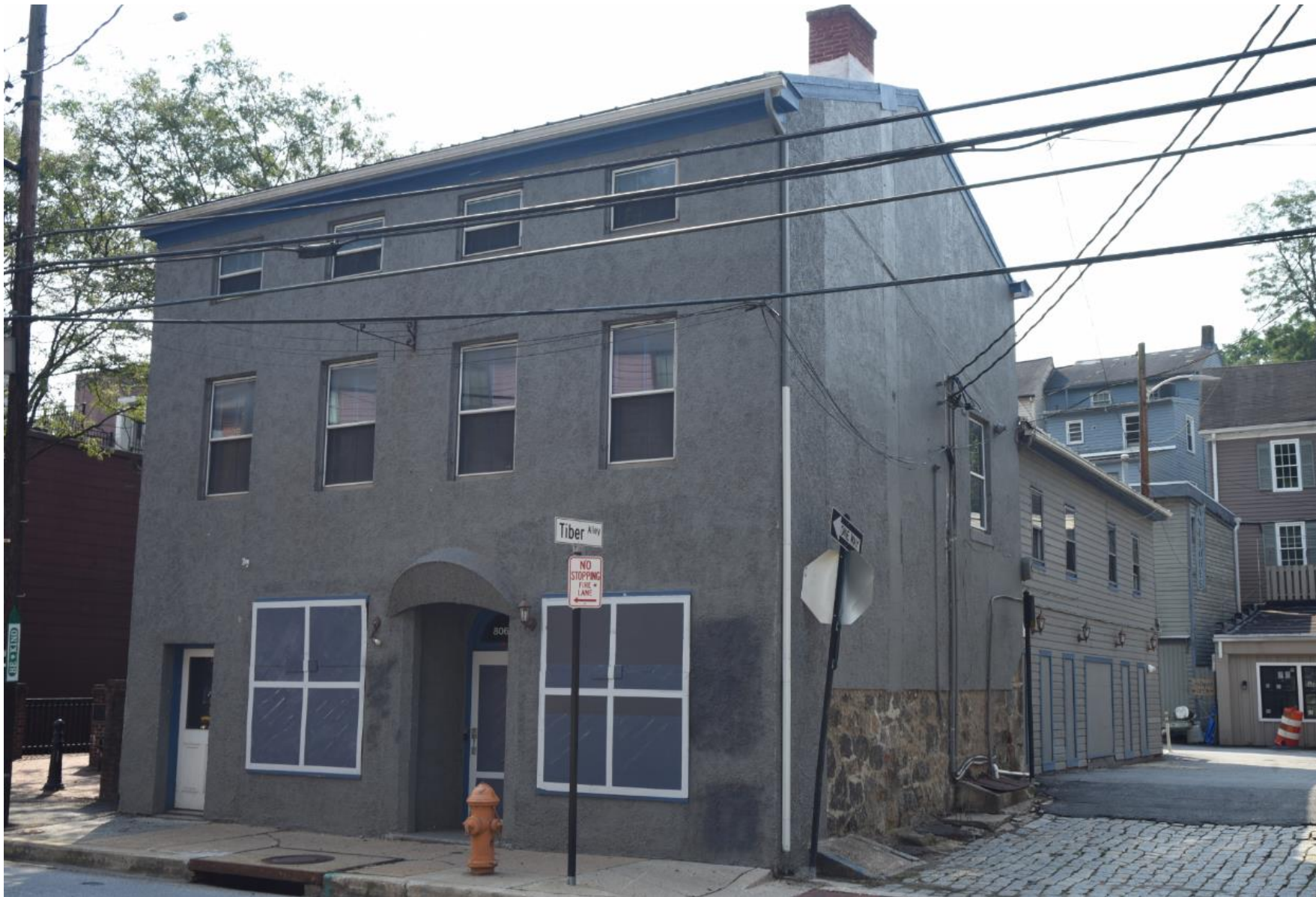
8069 Main Street front and west elevation adjacent to Tiber Alley.
