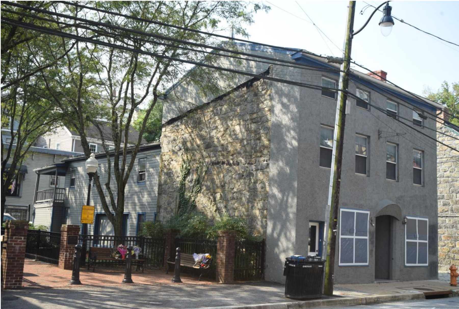
8069 Main Street front and east elevation adjacent to Tiber Park.
