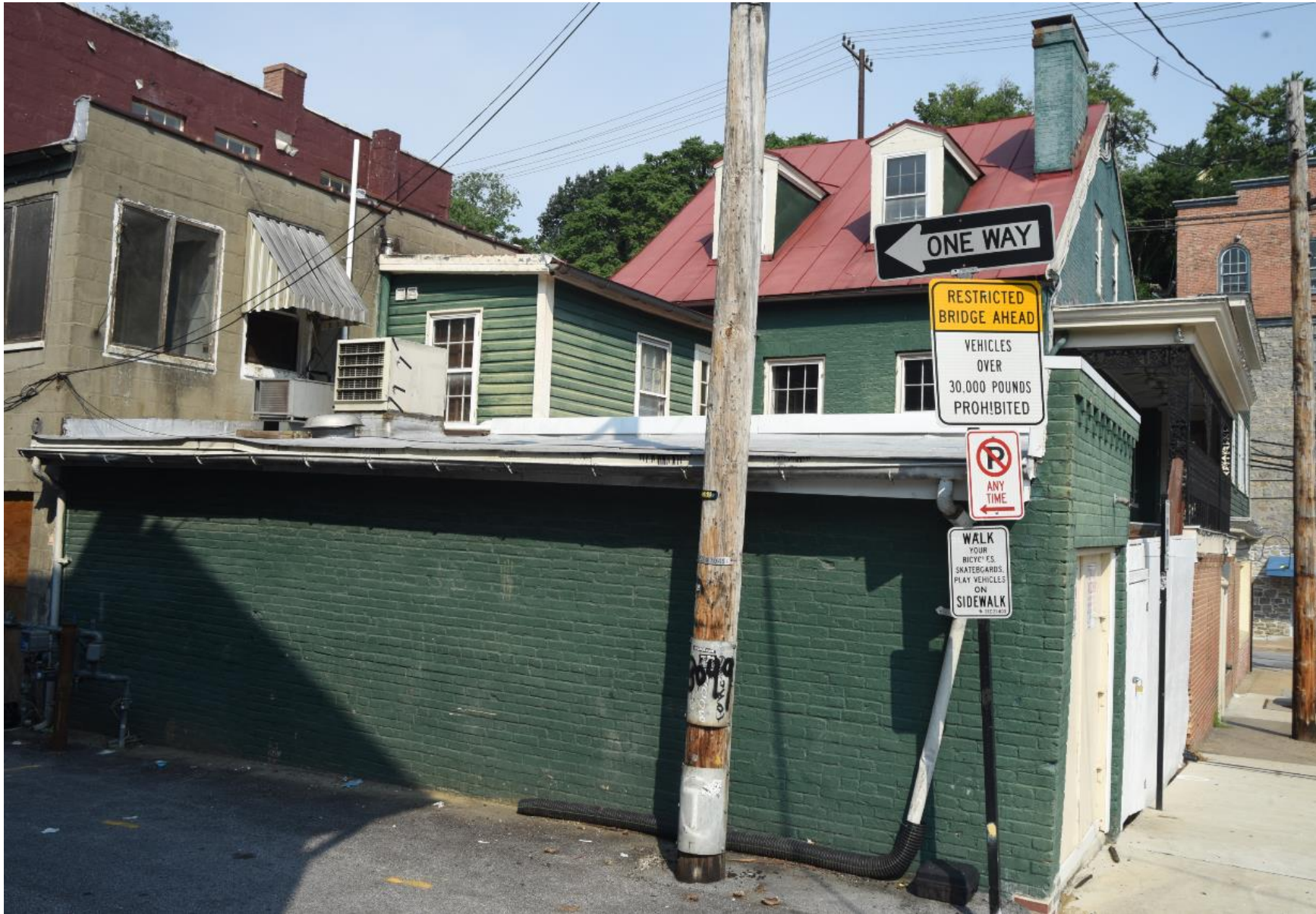
8049 Main Street - Rear of building along Tiber Alley
