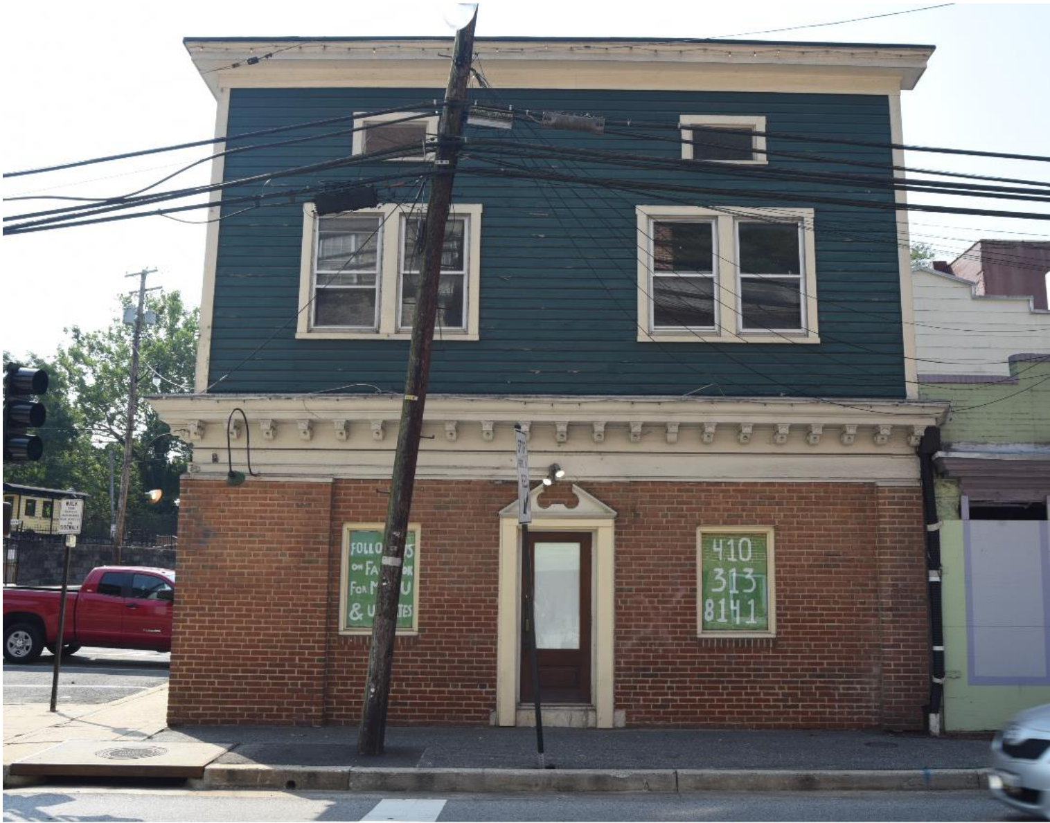
8049 Main Street front façade along Main Street
