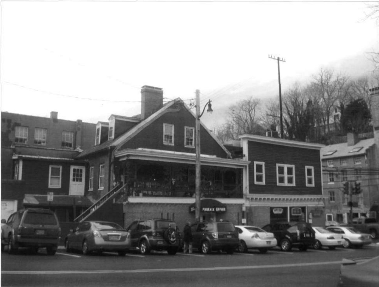
HO-330 Phoenix Emporium (P. Valmas Building, George Goeller Building) 8053 Main Street (MD 144), Ellicott City Photo by Jennifer K. Cosham, 12/5/2012 East elevation
