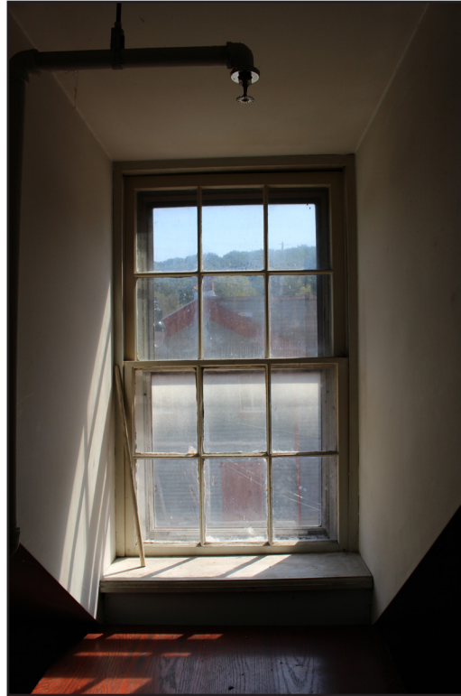
Figure 9: Six-over-six wood window in the attic. Tracerics, 2020
