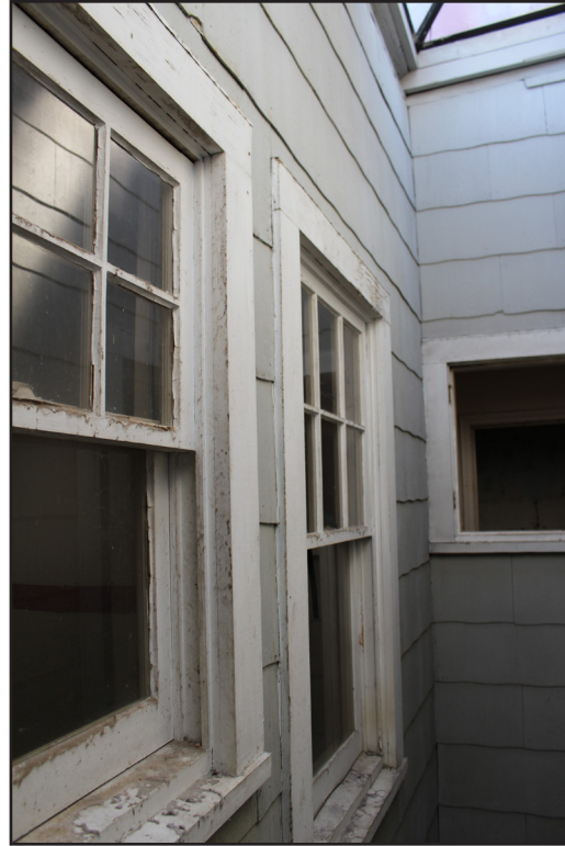
Figure 15: Wood windows and steel skylight. Tracerics, 2020
