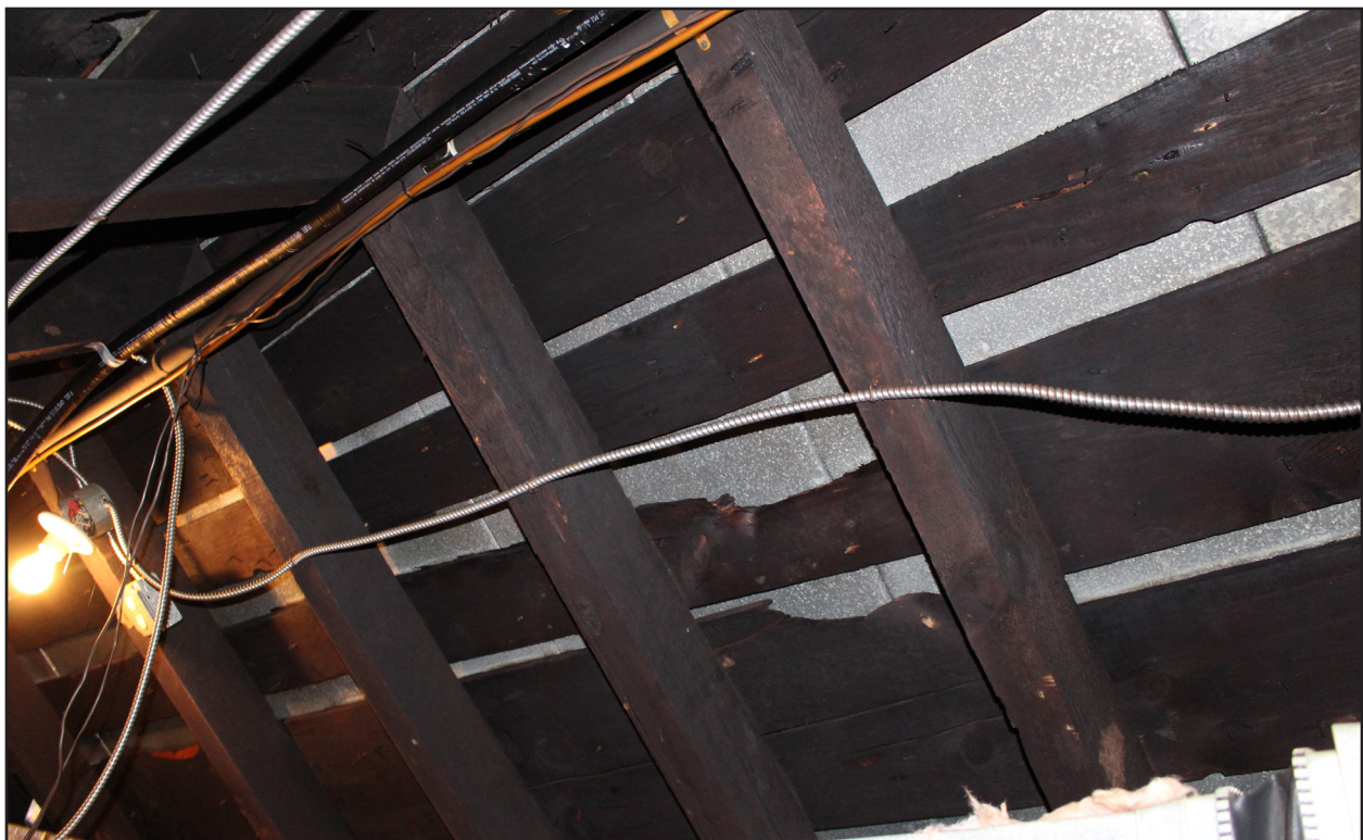
Figure 10: Wood roof rafters. Tracerics, 2020
