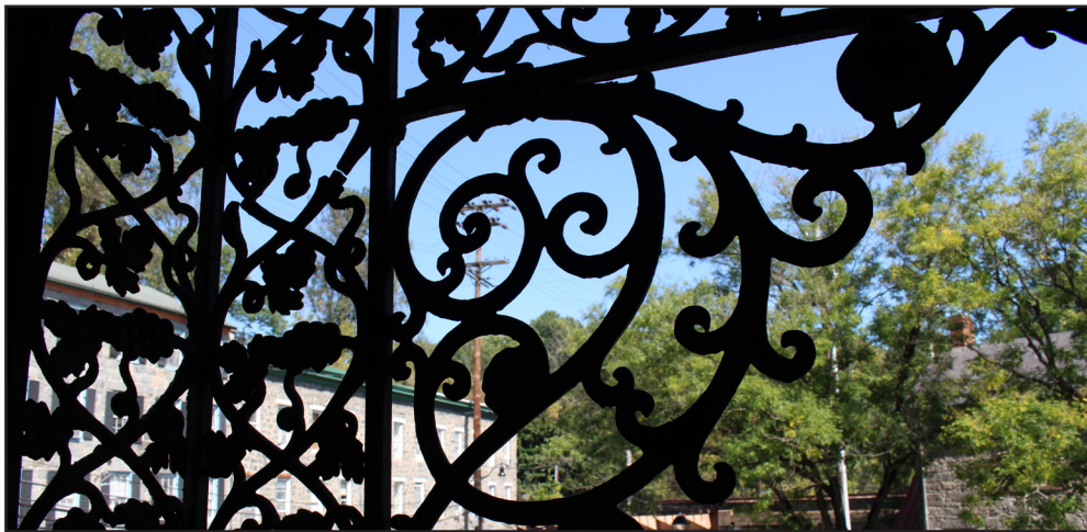
Figure 5: Detail of iron railing. Tracerics, 2020
