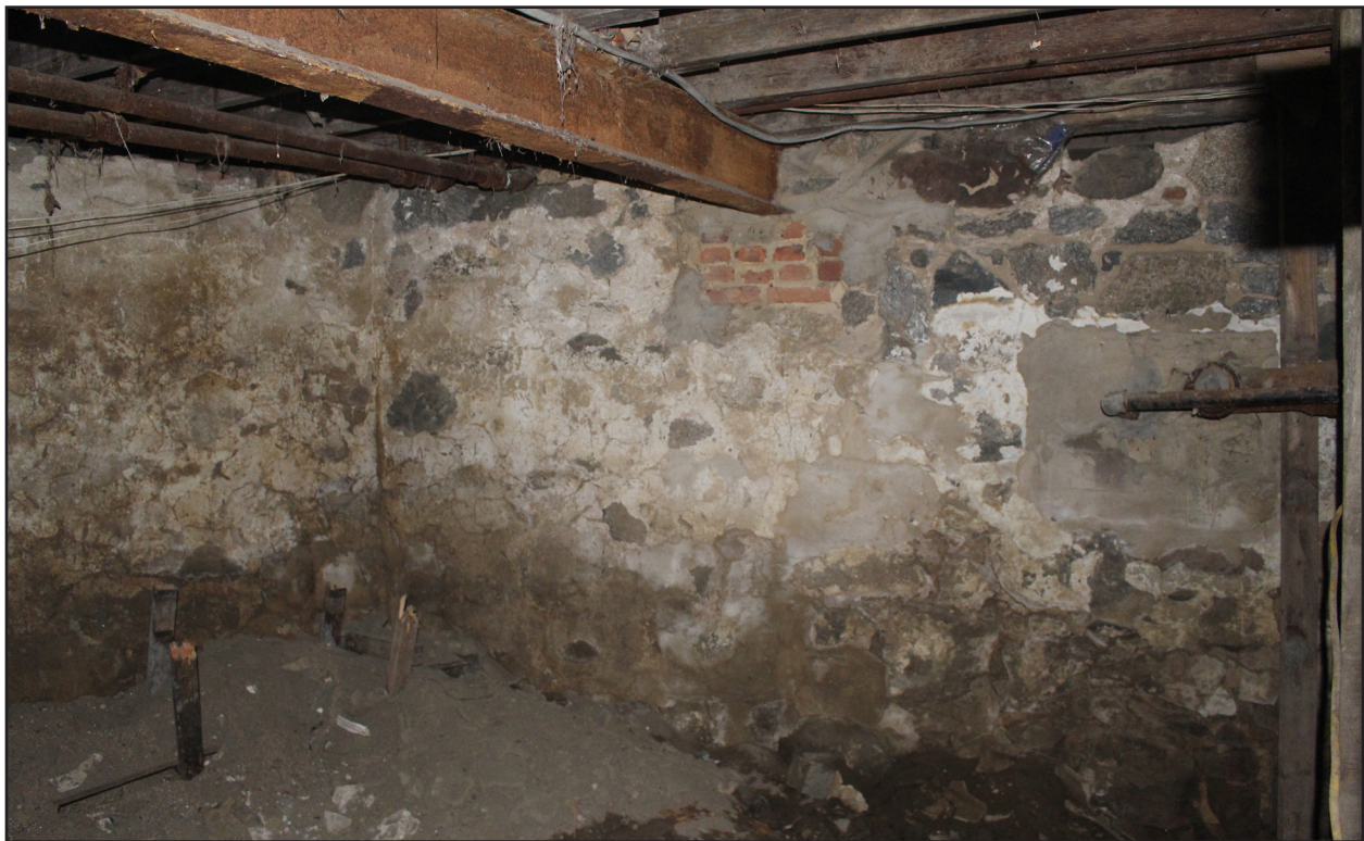
Figure 16: Fieldstone walls of the basement. Tracerics, 2020
