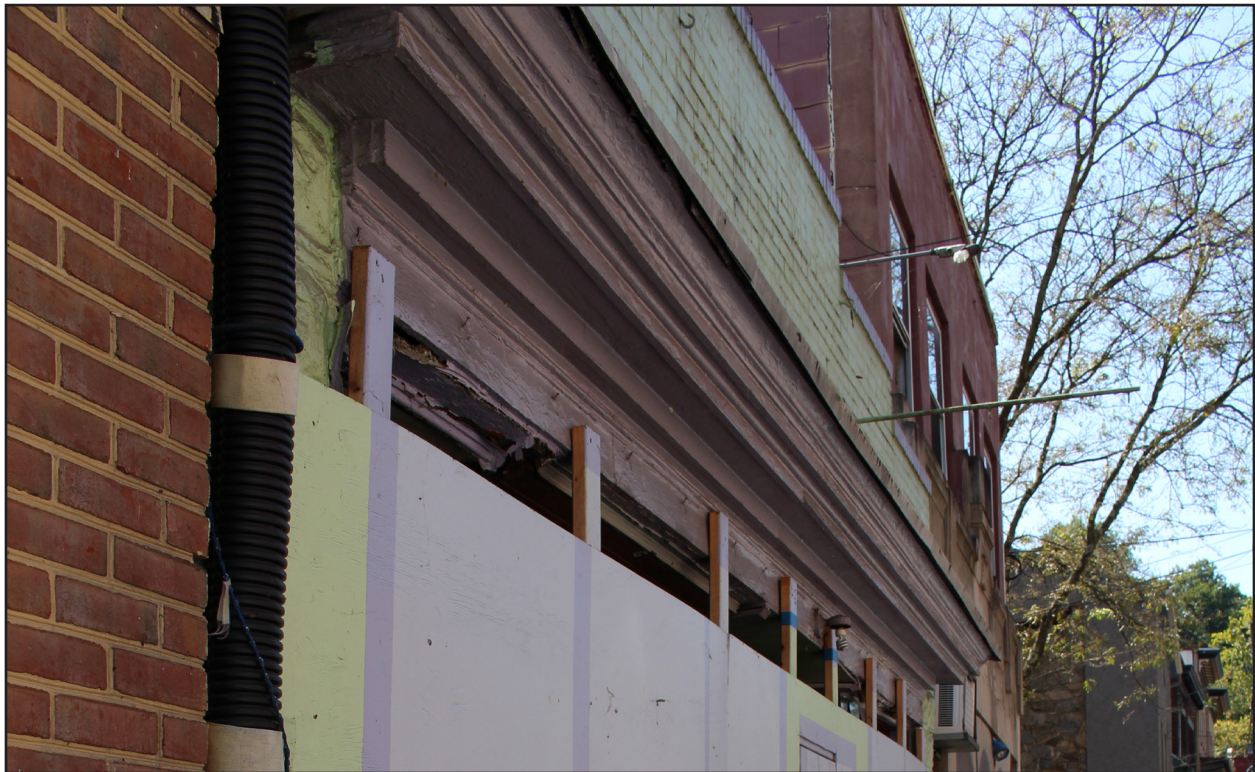
Figure 13: Wood cornice. Tracerics, 2020
