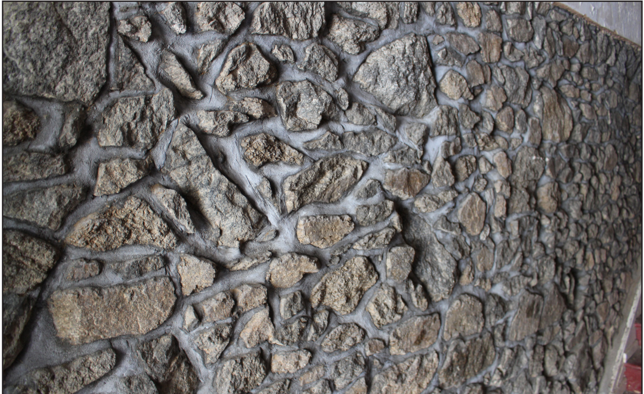
Figure 32: Stone wall. Traceries, 2020
