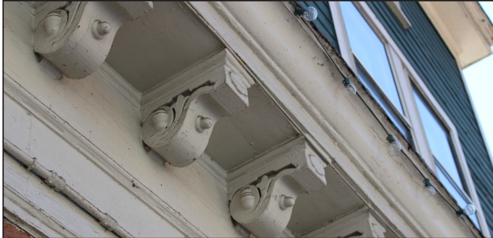
Figure 4: Detail of cornice. Tracerics, 2020
