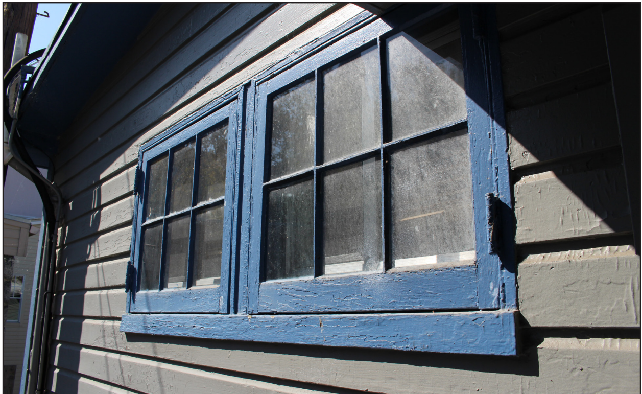
Figure 29: Wood windows. Tracerics, 2020
