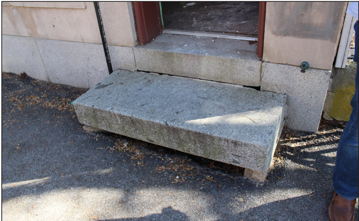
Figure 21: Granite base and entrance step. Tracerics, 2020
