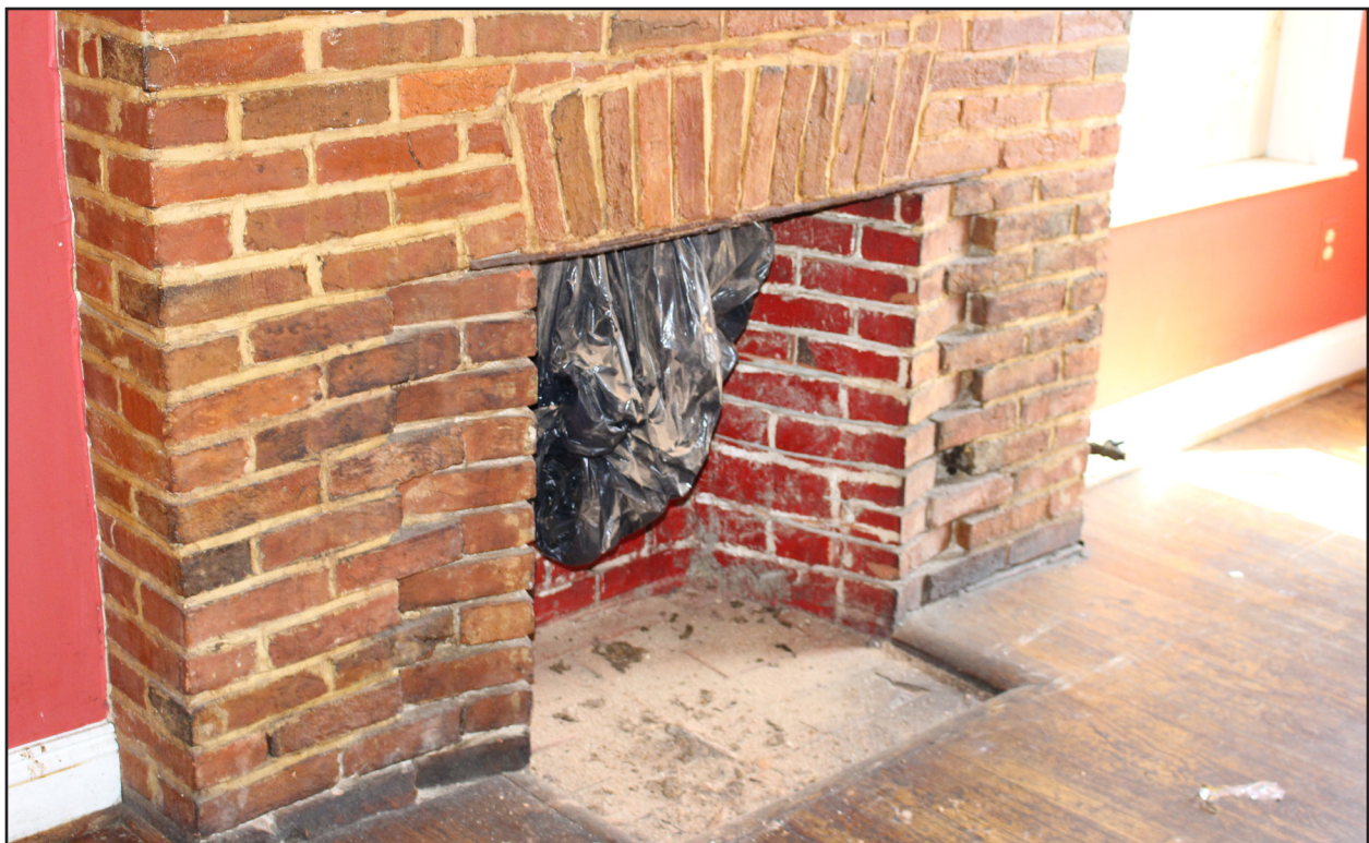
Figure 8: One of the two remaining chimney stacks in the building. Tracerics, 2020
