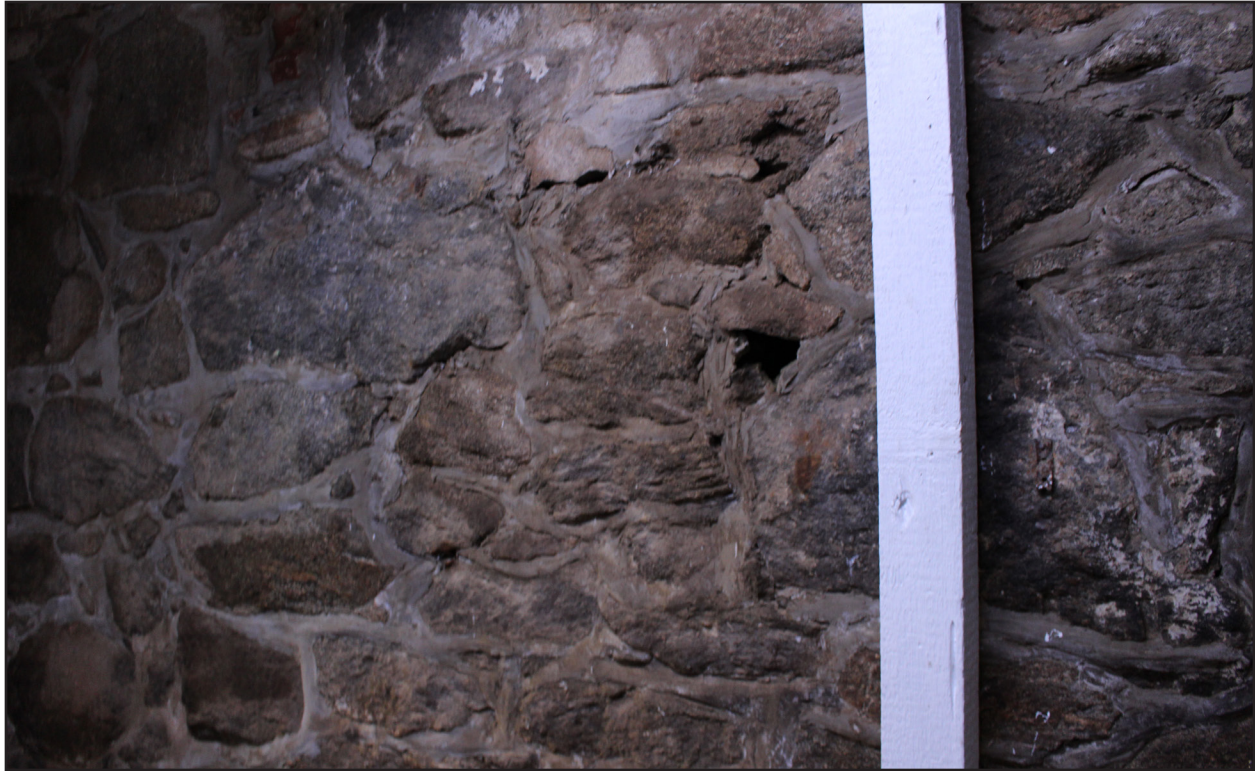
Figure 7: Fieldstone walls of the basement. Tracerics, 2020
