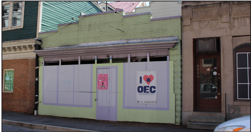
Figure 11: Facade 8055 Main Street. Tracerics, 2020
