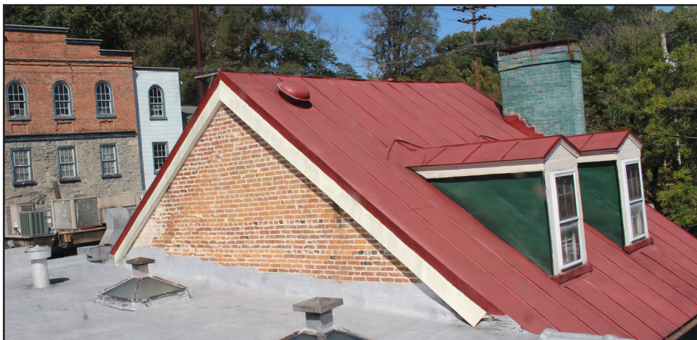
Figure 6: Standing seam metal roof. Tracerics, 2020
