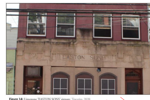
Figure 14: Exterior view of the building facade. Tricor, 2020
