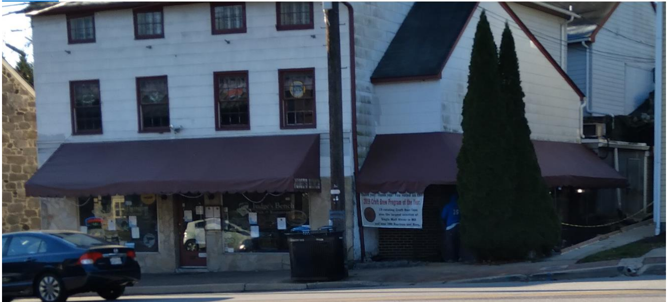
Figure 9 - Existing conditions. Awning on right side to be replaced. Front awning to remain.
