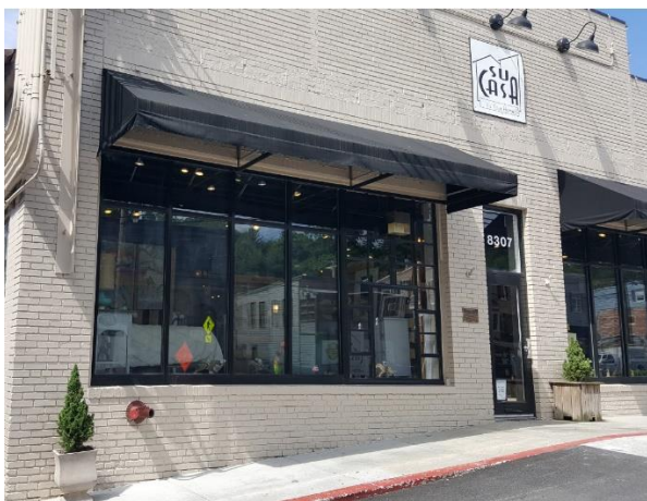
Figure 10 - Example of properly scaled awning.
