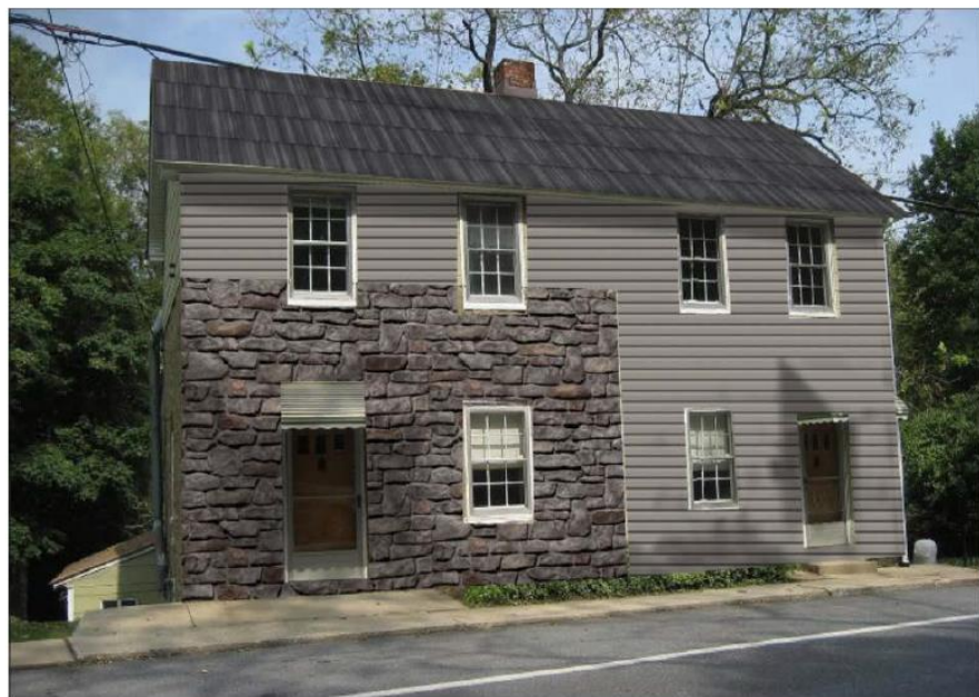
Figure 2 - Rendering of proposed alterations with solar shingles, restored gray siding and gray repointed mortar.
