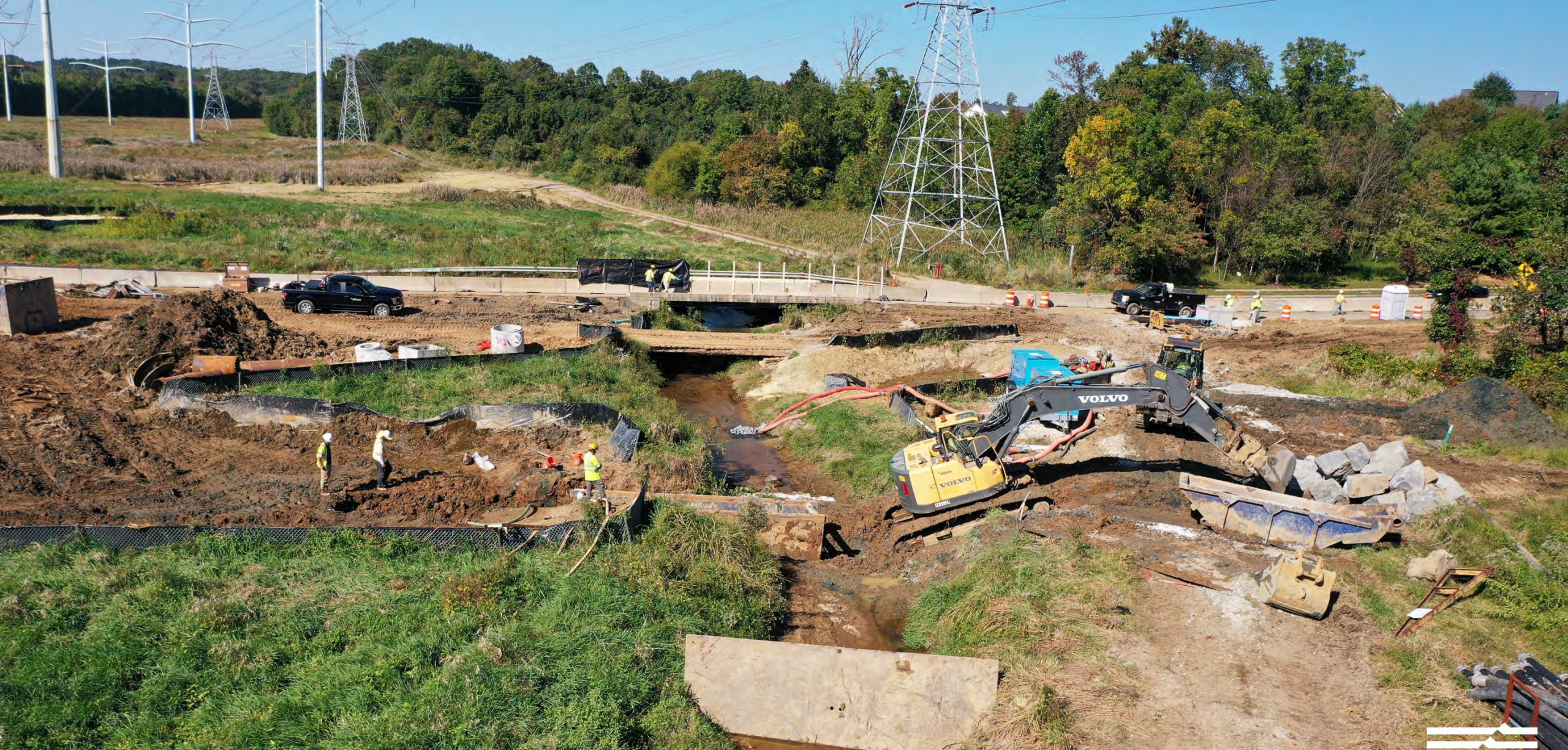
Stephens Road Improvements, Howard County, Maryland October 7, 2020, Day 106 of Project
