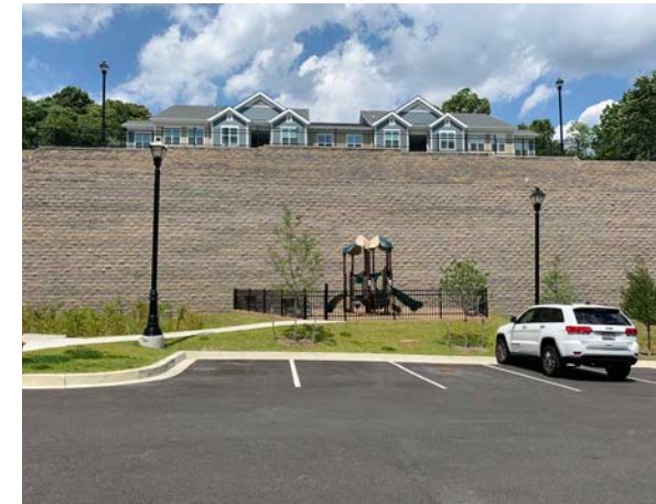
Figure 23: Architecture Not Responding to Overall Site
