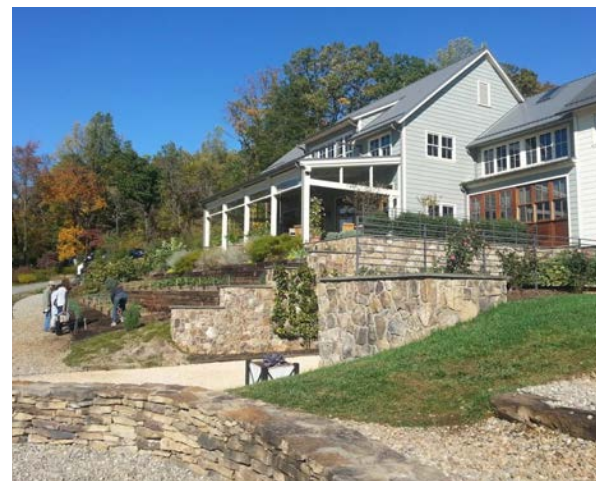
Figure 22: Site Design to Fit Architecture (Middle), Architecture Integrated into Site Design (Bottom)
