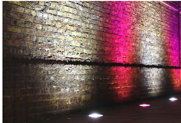
Figure 142: Wash Lighting Can Highlight Feature Walls, Credit: Nicobobinus Creative Commons
