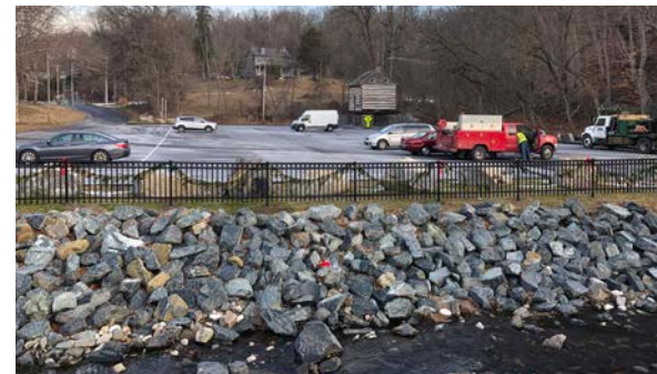
Figure 71: Boulders and Fencing Were Placed Between Lot F and the Stream Channel as Part of the Parking Lot's 2019 Reconfiguration.
