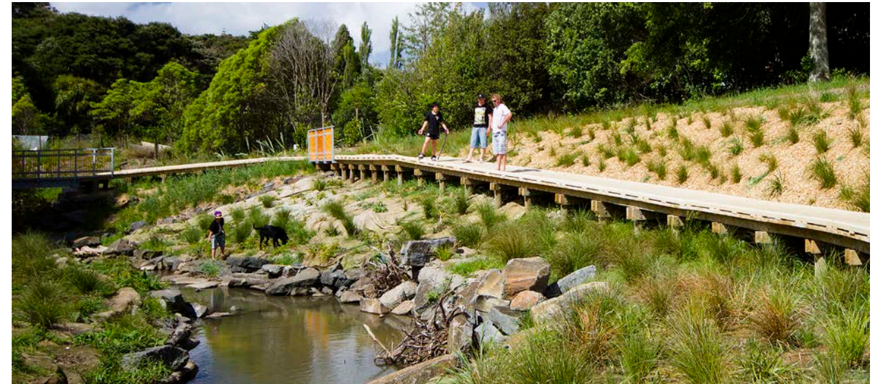
Figure 52: La Rosa Reserve Stream Daylighting Project in New Zealand, Credit: Boffa Miskell, Photographer: Claire Hamilton
