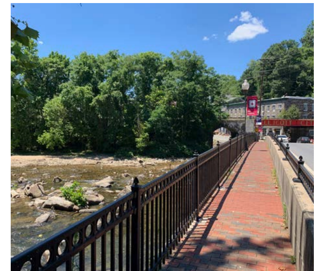
Figure 129: Opportunity to Enhance the Gateway Experience by Opening Views to the B&O Museum from the Patapsco River Bridge
