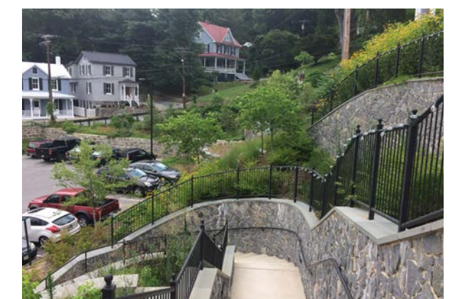
Figure 208: The Lot E Staircase Creates a Memorable Link Between the Courthouse Area and Main Street
