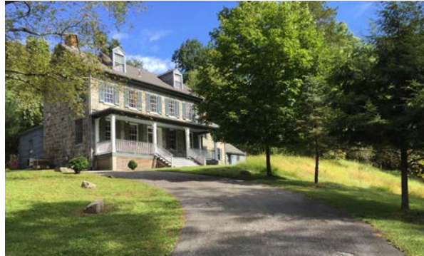
Figure 178: The Bernard Fort House has an Inviting Open Space that can be Viewed from Lot F
