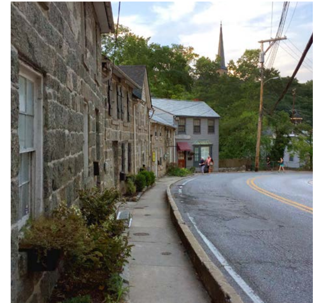
Figure 69: Narrow Sidewalk along Tonge Row Contribute to the Character of Ellicott City
