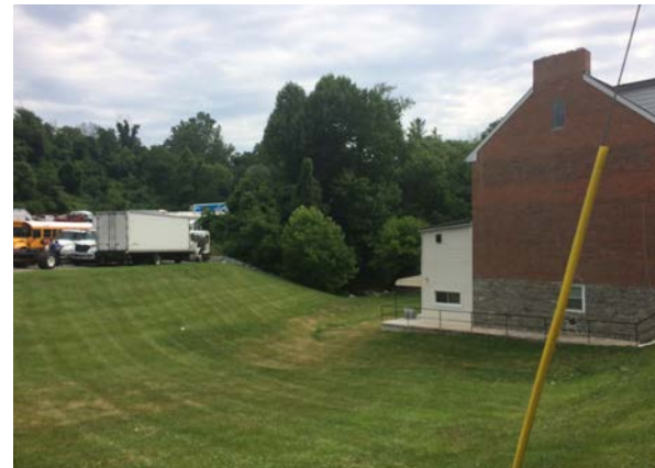
Figure 200: Existing Conditions at the West End Service Site, Hudson Branch is Currently Culverted Underneath the Site
