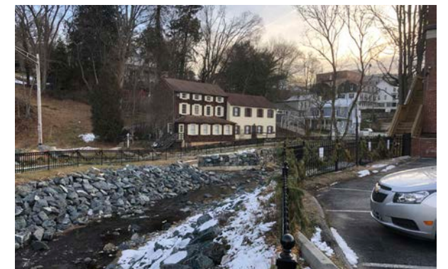
Figure 47: Daylighted Section of the Hudson Branch in Lot F After the Reconstruction Following the 2018 Flood
