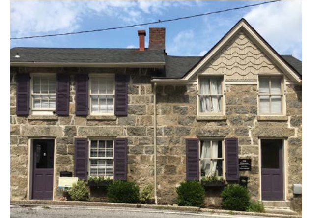
Figure 27: Rehabilitated Tonge Row Facades as part of Howard County Facade Improvement Program
