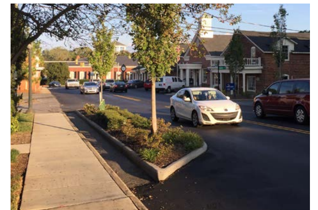
Figure 109: Modest ESD Practices Can Serve as Demonstration Projects in Lower Main
