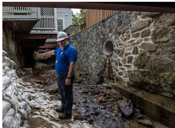
Figure 143: Character of Existing Stone Channel Walls
