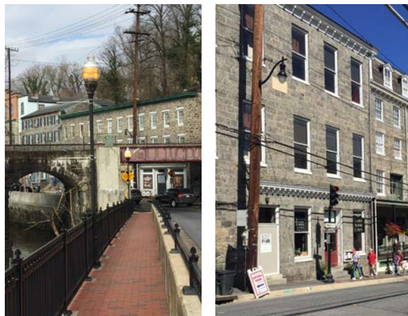
Figure 101: Existing Ornamental Lighting
